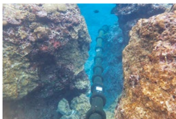
▲ Tokashiki Island submarine cable installation
