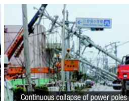
Continuous collapse of power poles
