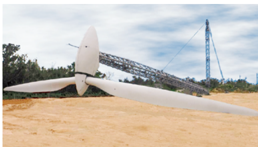
▲ Tarama Tilttable Wind Power Generation System/tilting state
