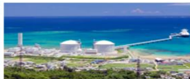
Yoshinoura Thermal Power Plant
