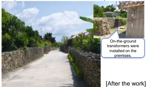
[Case example] The removal of utility poles in locations where there is no pedestrian road and no ground equipment can be installed on the road (Taketomicho, Taketomi Island)
