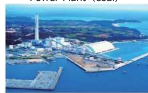
Kin Thermal Power Plant (coal)
