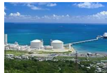
Yoshinoura Thermal Power Plant (LNG)
