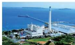
Gushikawa Thermal Power Plant (coal)
