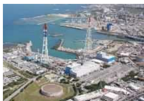
Makiminato Thermal Power Plant (oil)
