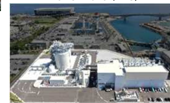
Makiminato Gas Engine Power Plant (LNG)
