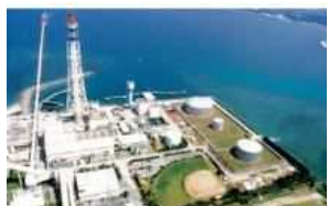
Ishikawa Thermal Power Plant (oil)
