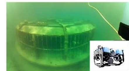
<Water inlet inspection by underwater drone>
