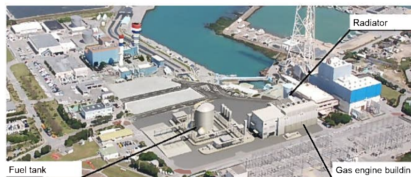
Image of the power station
