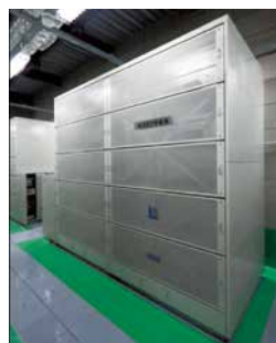
Miyako Island Mega Solar Power Demonstration Research Facility (NaS battery)
