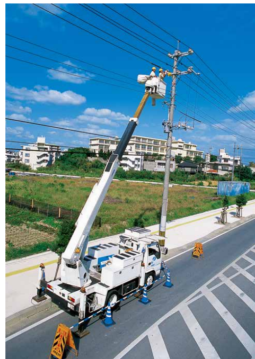
Distribution line maintenance
