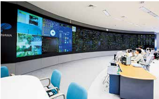
Load dispatching center
