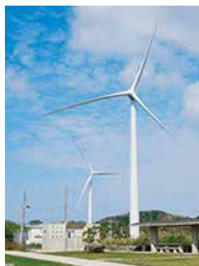
Ogimi Wind Power Generation Demonstration Research Facility
