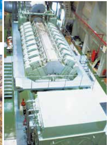
Ishigaki No. 2 Power Plant (diesel generator)
