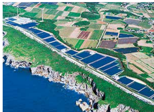
Miyako Island Mega Solar Power Demonstration Research Facility
