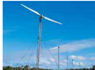
Tilttable wind turbine power plant (275 kW×5 turbines) in Tonga
