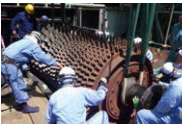
Gas turbine inspection at the Makiminato Thermal Power Plant: Okinawa Plant Kogyo Co., Ltd.
