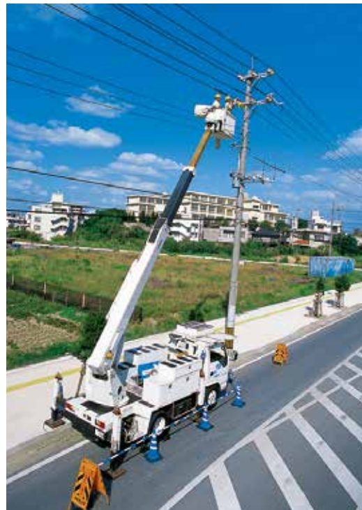
Distribution line maintenance
