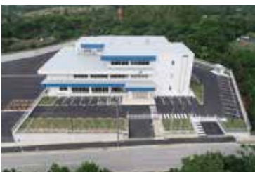
Okiden Nago Building, OEPC's new office building: Okiden Kaihatsu Co., Inc. (Design: Okinawa Enetech Co., Inc.; Construction: Okidenko Co., Inc.)
