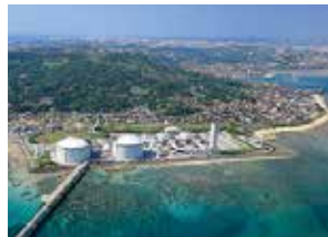
Yoshinoura Thermal Power Plant
