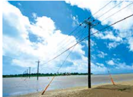
Power distribution line continuing through to Yubu Island
