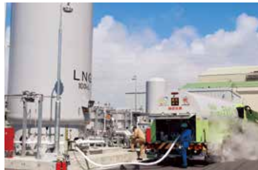
Unloading operation at a natural gas supply center
