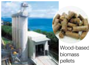
Wood-based biomass distribution facility
