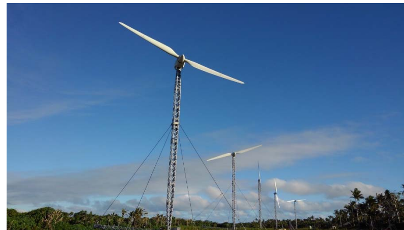
▲ Tiltable wind power generators at the Kingdom of Tonga.
