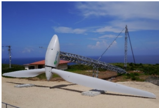
▲Aguni tiltable wind power generators when tilted
