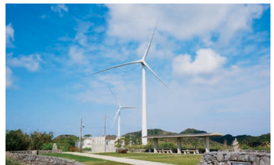
Ogimi Wind Power Generation Demonstration Research Facility
