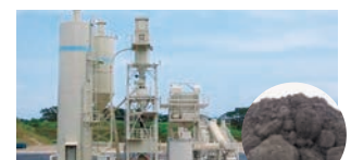
Plant producing alternative materials from the waste
