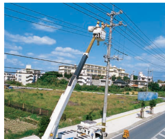
Distribution line maintenance
