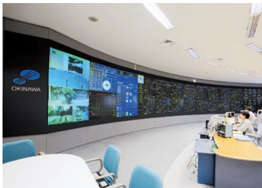
Load dispatching center
