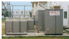
Ice-storage air conditioning systems
