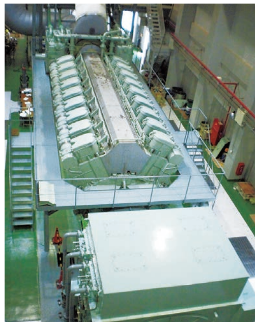
Ishigaki No. 2 Power Plant (diesel generator)
