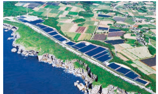
Miyako Island Mega Solar Power Demonstration Research Facility
