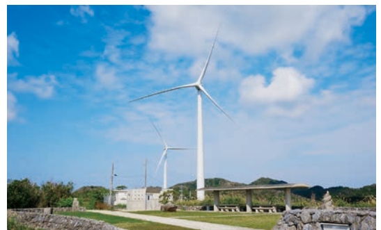
Ogimi Wind Power Generation Demonstration Research Facility
