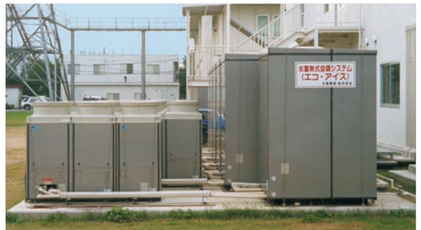
Ice-storage air conditioning systems
