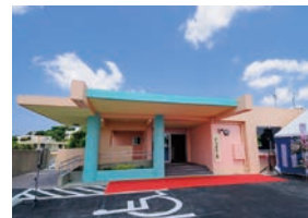
OEPC donated funds for construction of Family House, for accommodation of parents and other relatives visiting patients at Nanbu Prefectural Medical Center, a children's care facility.
