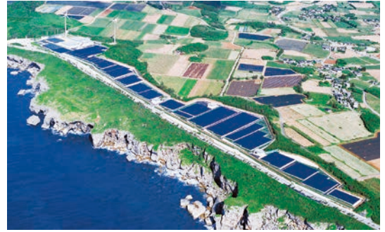
Miyako Island Mega Solar Power Experimental Research Facility
