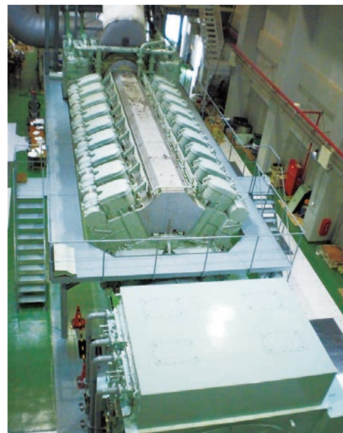
Ishigaki No. 2 Power Plant (diesel generator)
