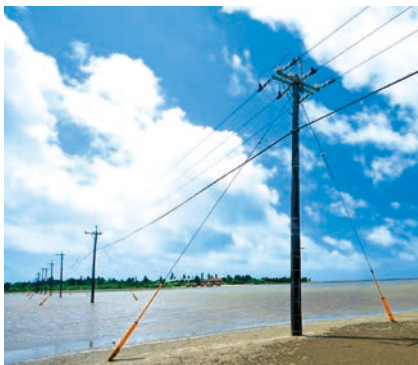
Power distribution line continuing through to Yubu Island
