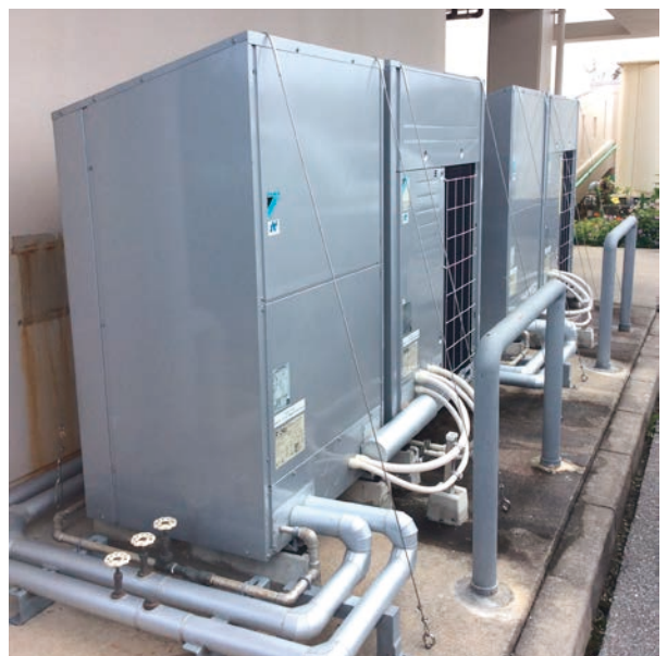
Commercial heat-pump hot-water supply system
