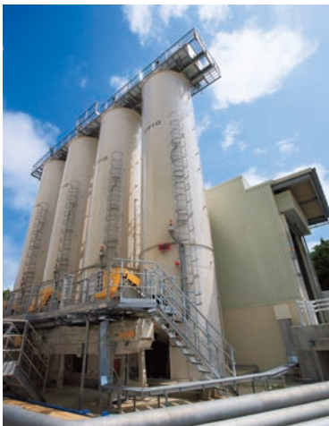
Biomass co-firing system
