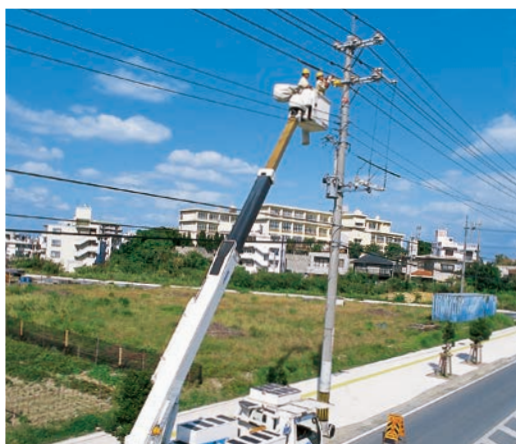
Distribution line maintenance
