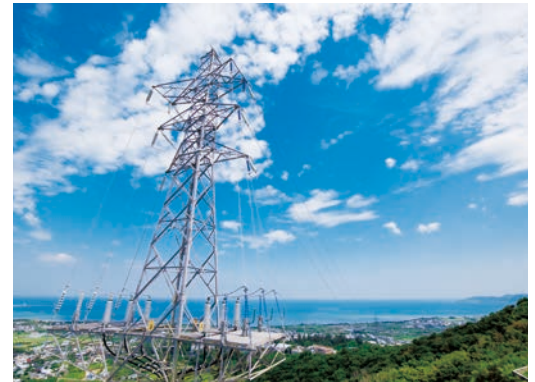
Transmission and distribution facility
