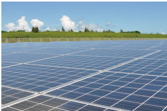
Solar power generation system on Tarama Island
