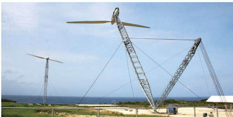
Retractable wind turbines at Hateruma Island
