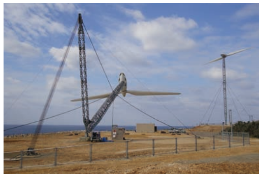
Retractable wind turbine (Minami-Daito Island)
