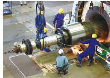
Turbine check at Kin Thermal Power Plant (Okinawa Plant Kogyo Co., Inc.)
