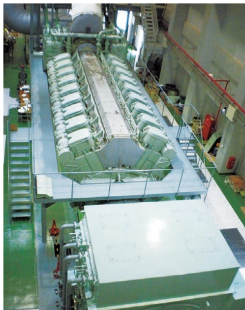
Ishigaki No. 2 Power Plant (diesel generator)
