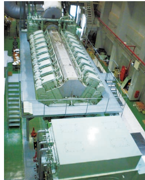
Ishigaki No. 2 Power Plant (diesel generator)
