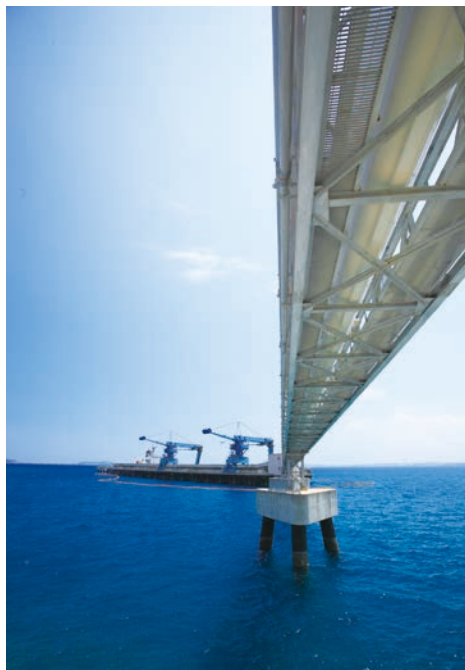
Kin Thermal Power Plant
