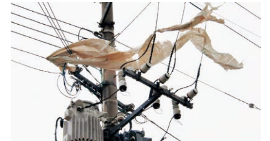
Damage due to flying debris
