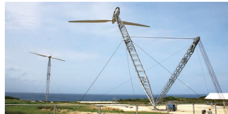
Retractable wind-power generator at Hateruma Island
