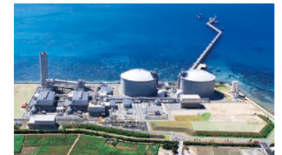
Yoshinoura Thermal Power Plant
