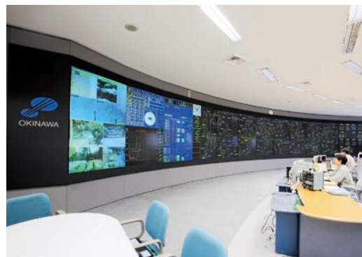
Load dispatching center
