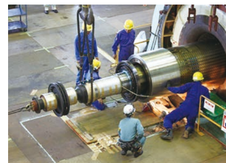
Turbine check at Kin Thermal Power Plant (Okinawa Plant Kogyo Co., Inc.)
