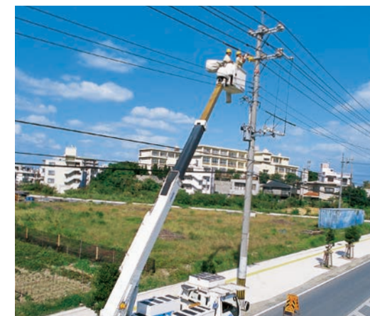
Distribution line maintenance
