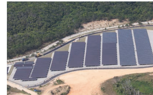
Abu Mega Solar Power Experimental Research Facility
