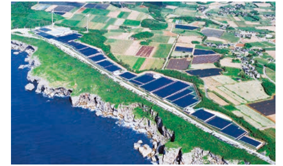
Miyako Island Mega Solar Power Experimental Research Facility
