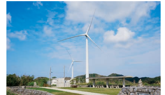
Ogimi Wind Power Generation Demonstration Research Facility
