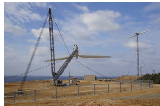
Retractable wind-power generator (Minami-Daito Island)
