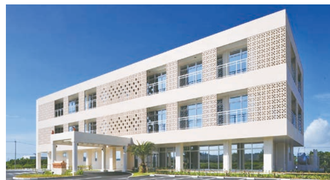
Building No. 2, Corporate Integrated Facility, Okinawa IT Shinryo Park (Okiden Kaihatsu Co., Inc.)
