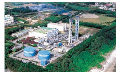
Green power plant (Ishigaki No. 2 Power Plant)
