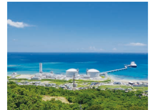
Yoshinoura Thermal Power Plant
