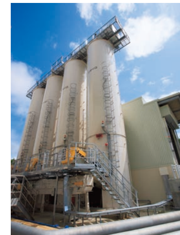
Biomass co-firing system
