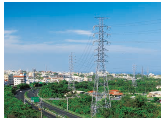
Transmission and distribution facilities
