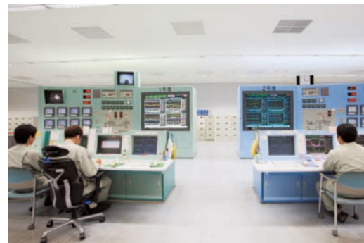
Kin Thermal Power Plant control room
