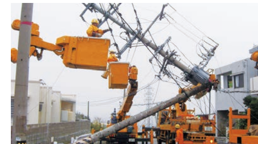
Electric power restoration operations
