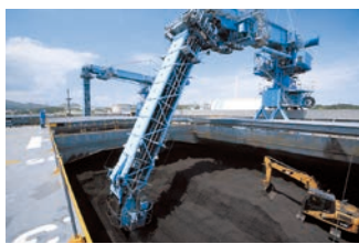
Unloading coal at Kin Thermal Power Plant
