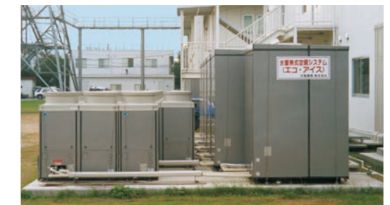
Ice-storage air conditioning systems
