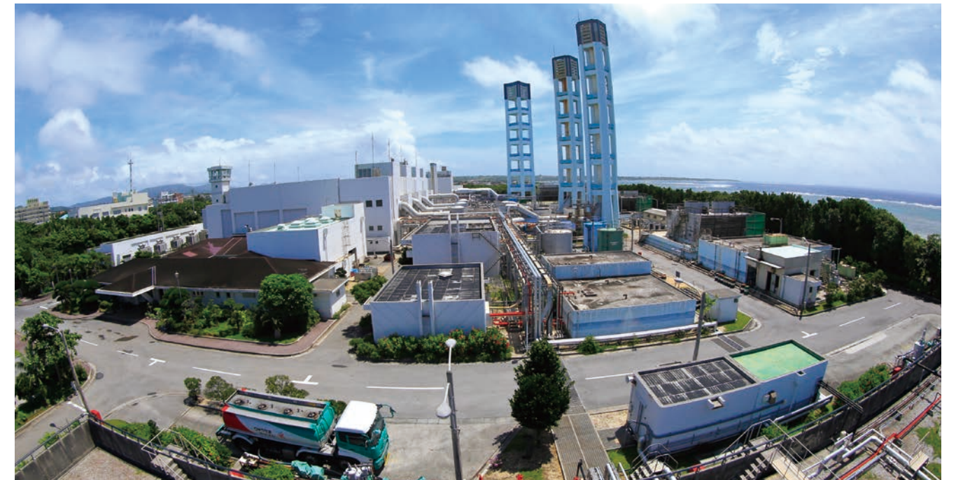
Ishigaki No. 2 Power Plant
