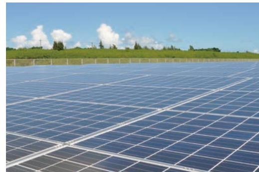
Solar power generation system on Tarama Island
