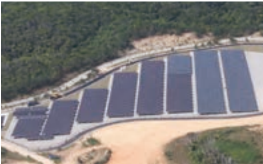
Abu Mega Solar Power Experimental Research Facility
