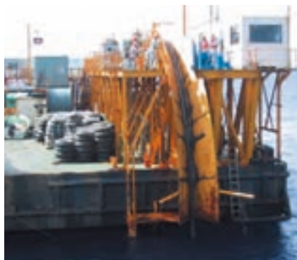
Laying submarine power cables
