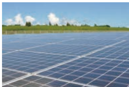
Solar power generation system on Tarama Island
