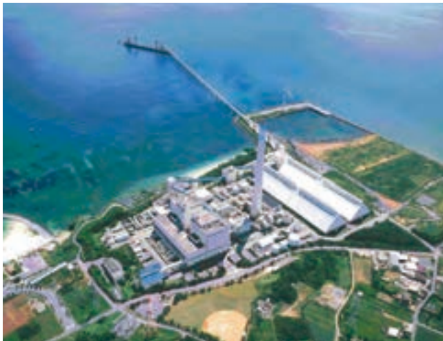
Gushikawa thermal power plant
