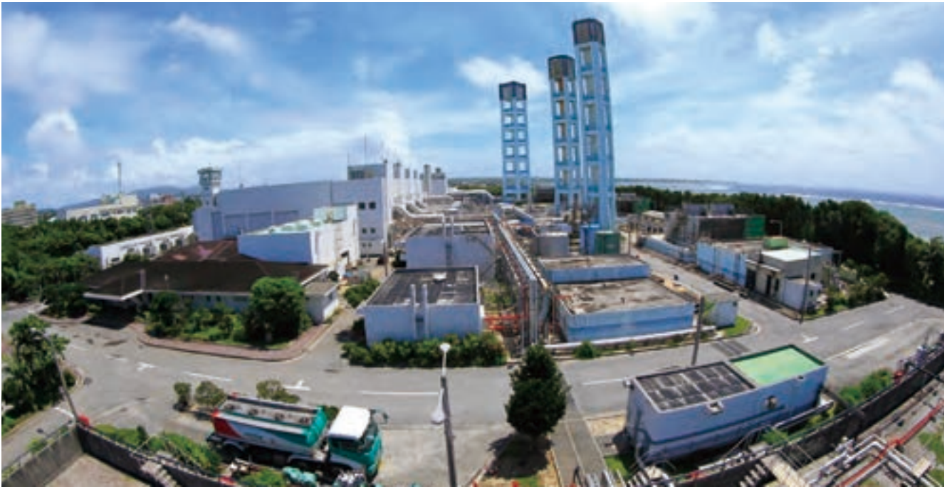
Miyako No. 2 internal combustion power station
