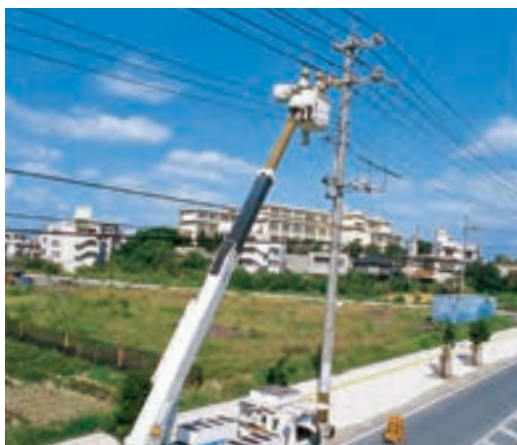
Maintenance of distribution lines
