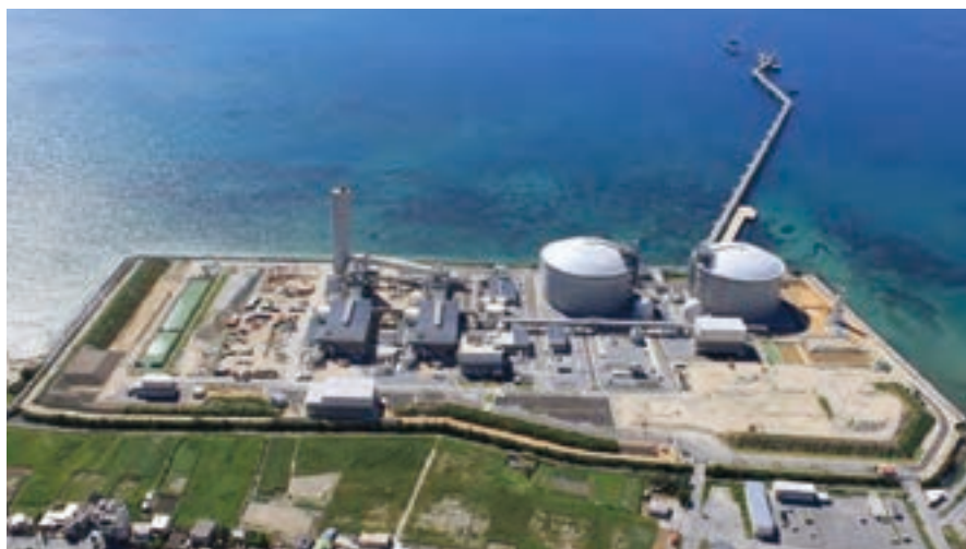
Yoshinoura thermal power plant during construction
