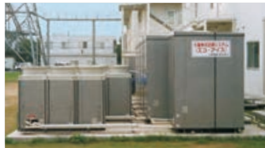
Ice-storage air conditioning systems
