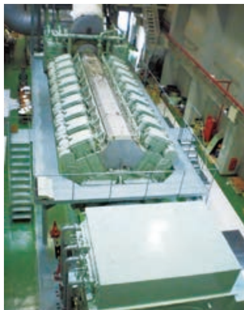
Ishigaki No. 2 Power Plant (diesel turbine)
