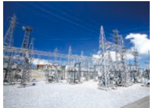
OEPC pylons in Okinawa
