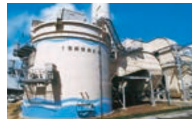
Environmental protection facilities at a power plant As part of an overall policy of removing harmful chemicals from smoke emitted by our power plants, they are equipped with desulfurization and denitrification equipment.
