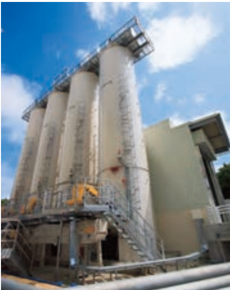
Biomass co-firing system
