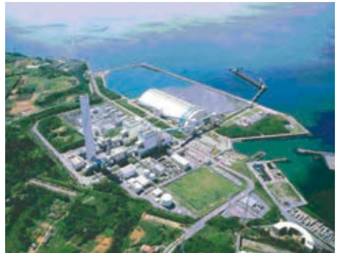
Kin thermal power plant
