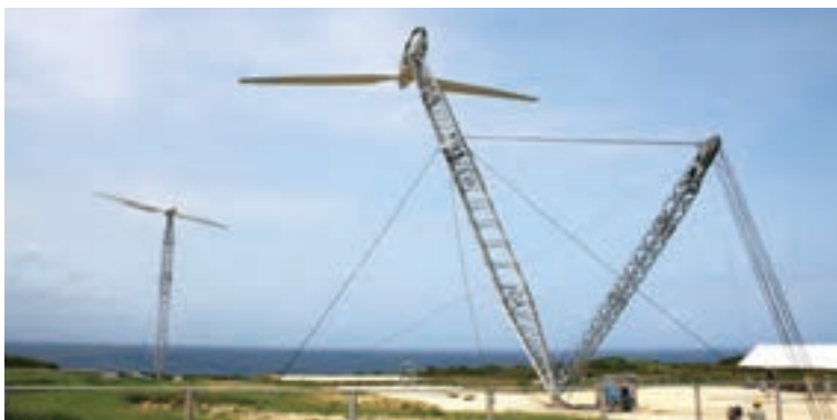
Retractable wind-power generator at Hateruma Island
