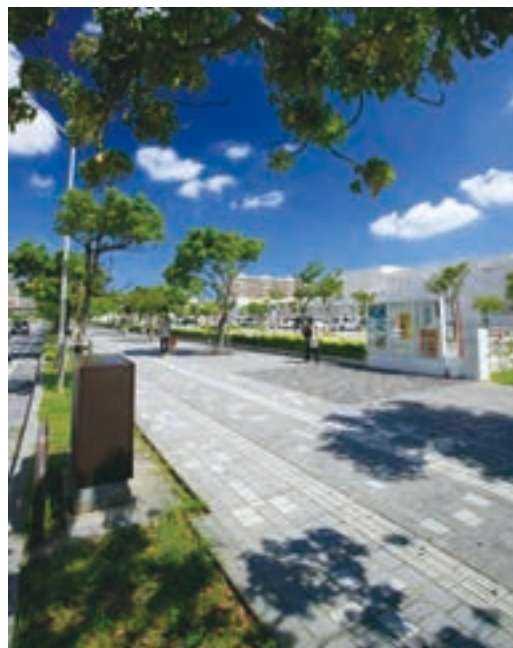
Street with underground power distribution lines
