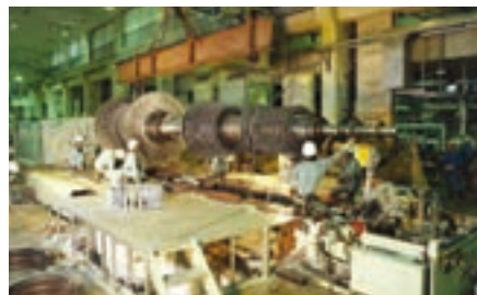
Staff from Okinawa Plant Kogyo Co., Inc. disassemble a turbine at Makiminato Thermal Power Plant for a regular inspection.
