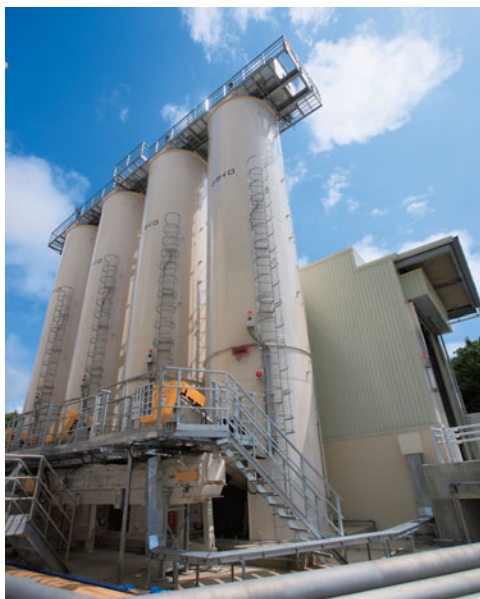
Biomass co-firing system
