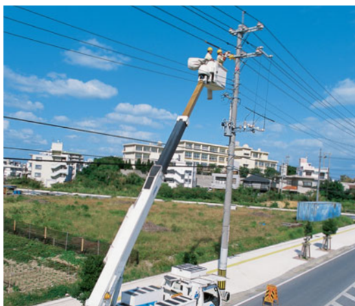
Maintenance of distribution lines
