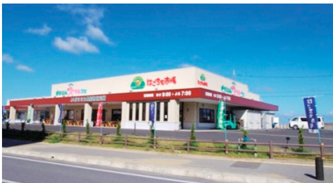
Ginowan Yui Marche: Built and maintained by Okiden Kaihatsu Co., Inc.
