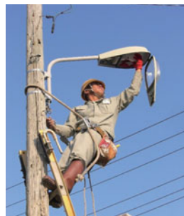
OEPC employees inspecting street lights
