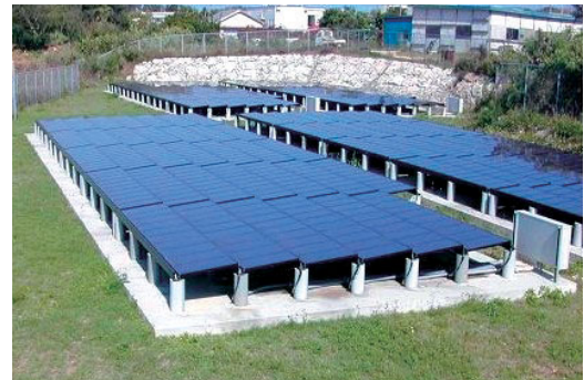
Solar power generation system on Kita-Daito Island
