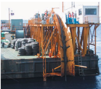
Laying submarine power cables
