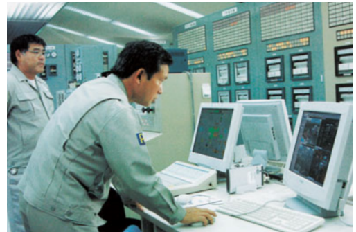
Remote monitoring of Ishigaki power plants
