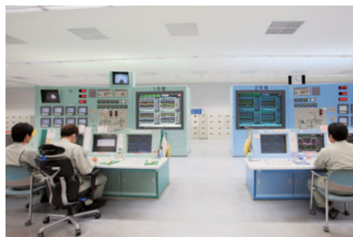
Kin Thermal Power Plant control room
