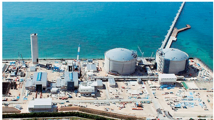
Yoshinoura thermal power plant during construction
