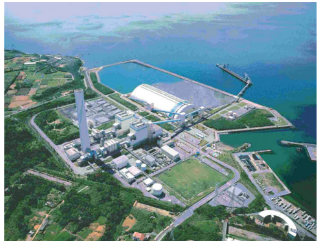
Kin thermal power plant
