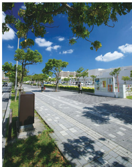
Street with underground power distribution lines
