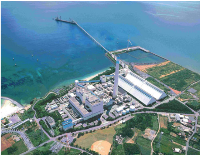
Gushikawa thermal power plant
