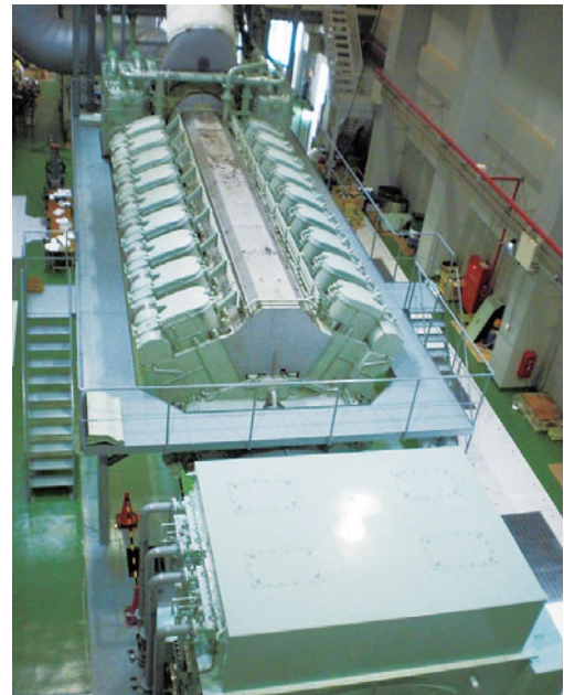
Ishigaki No. 2 Power Plant (diesel turbine)
