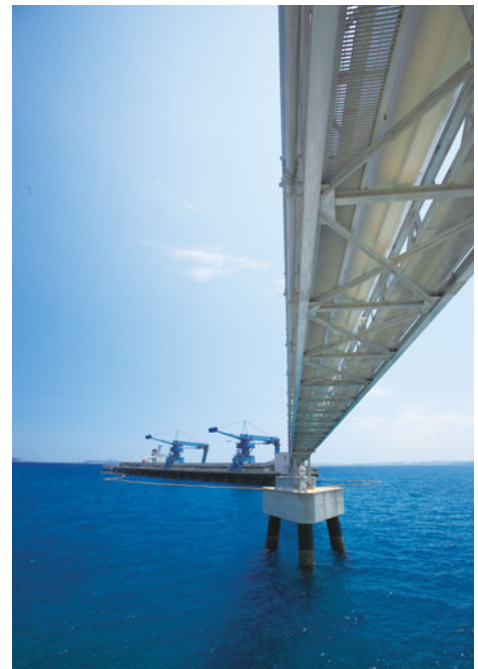
Kin thermal power station
