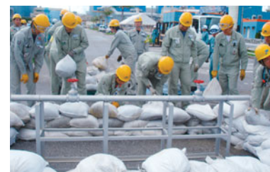
Stacking sandbags at Makiminato Thermal Power Plant
