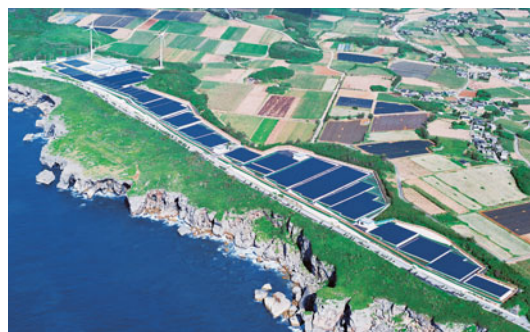
Solar power system on Miyako Island field test facility
