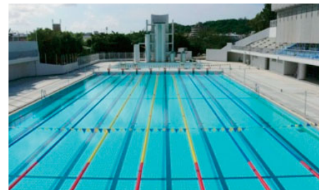
Repair works at Ounoyama Park swimming pool in Naha (Okidenko Co., Inc.)
