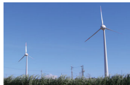
Wind power generators
