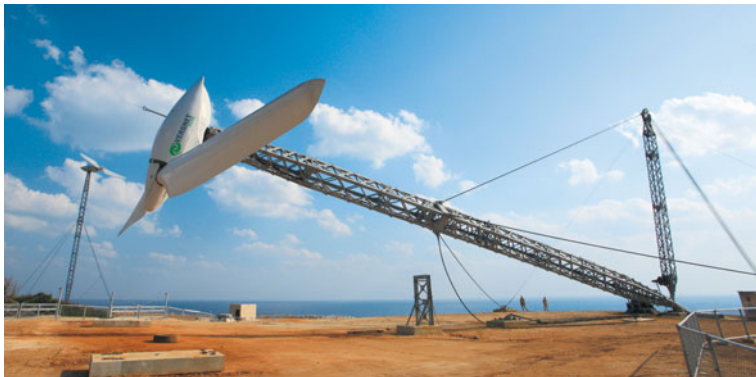
Retractable wind-power generator at Hateruma Island
