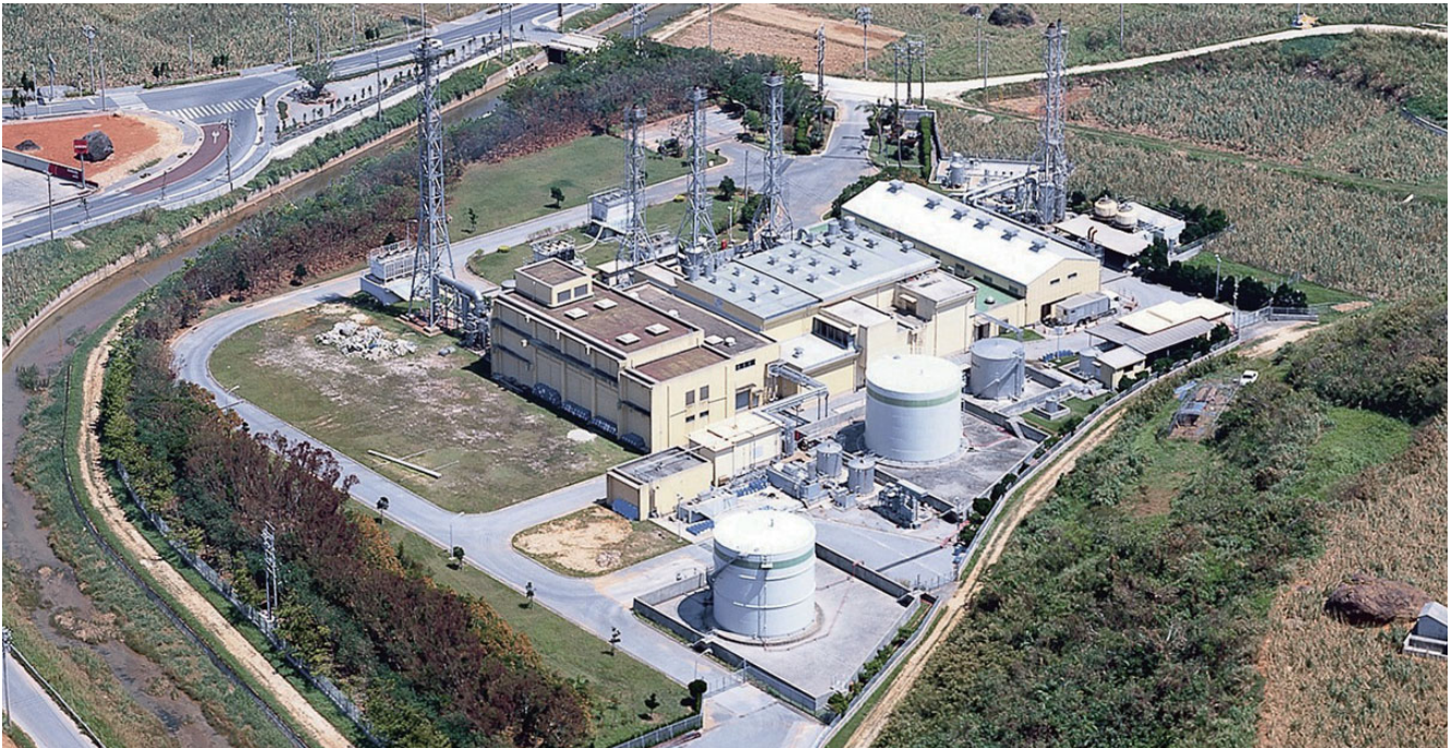
Kumejima power plant
