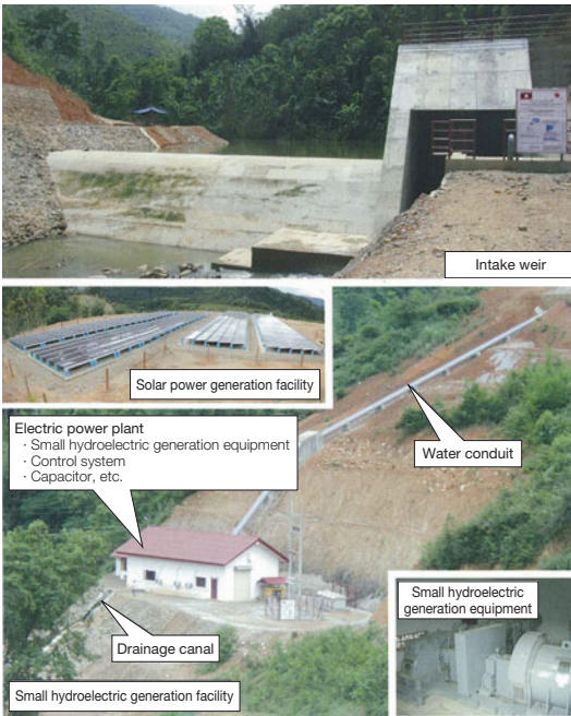
Solar power microgrid system (Laos)
