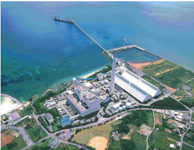
Gushikawa thermal power plant
