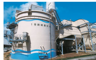
Environmental protection facilities at a power plant As part of an overall policy of removing harmful chemicals from smoke emitted by our power plants, they are equipped with desulfurization and denitrification equipment.
