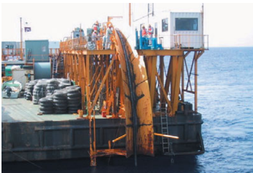
Laying submarine power cables
