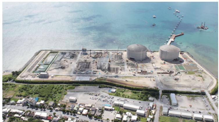
Yoshinoura thermal power plant during construction
