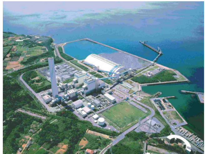
Kin thermal power plant
