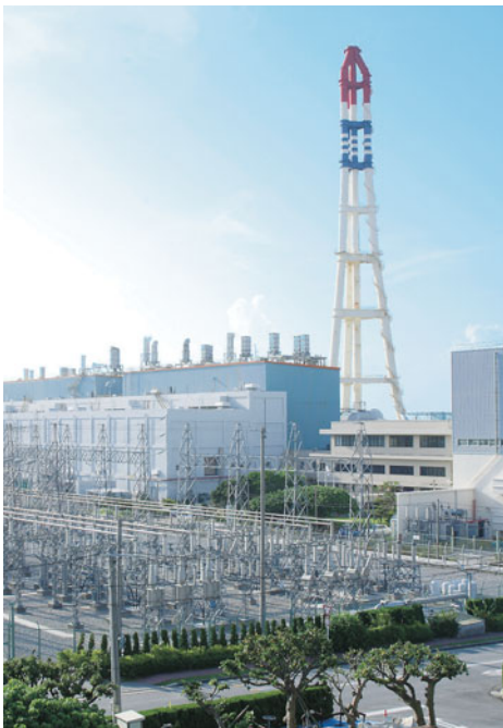
Makiminato thermal power station
