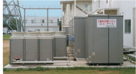
Ice-storage air conditioning systems
