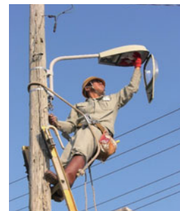
OEPC employees inspecting street lights
