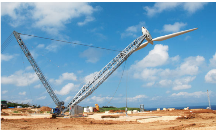
Retractable wind-power generator at Hateruma Island
