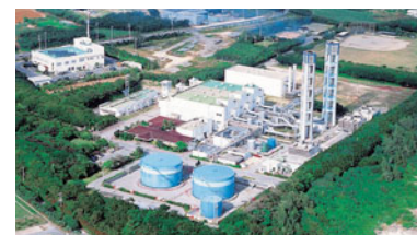
Ishigaki No. 2 Power Plant (diesel turbine plant surrounded by 90,000 native trees planted by the Company)
