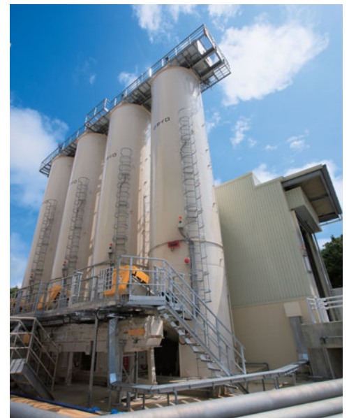
Biomass co-firing system
