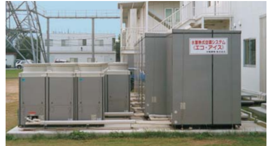
Ice-storage air conditioning systems
