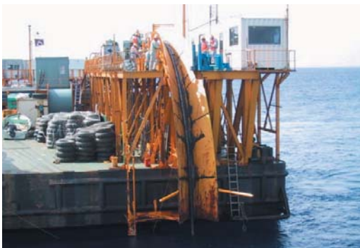
Laying submarine power cables
