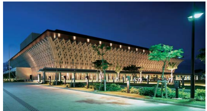
Okidenko Company Incorporated installed the exterior lighting for the National Theater Okinawa.
