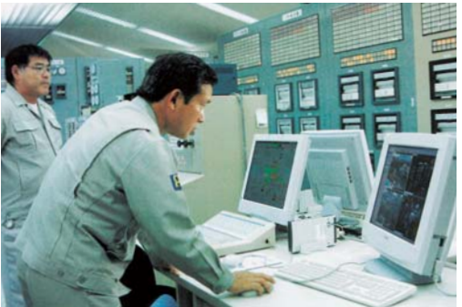
Remote monitoring of Miyako and Ishigaki power plants
