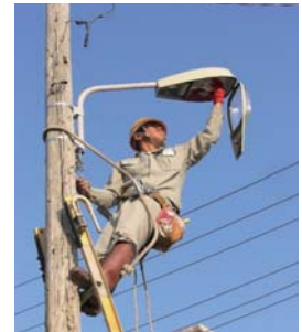
OEPC employees inspecting street lights
