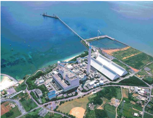
Gushikawa thermal power plant
