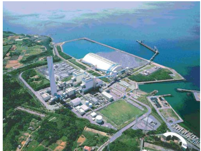
Kin thermal power plant
