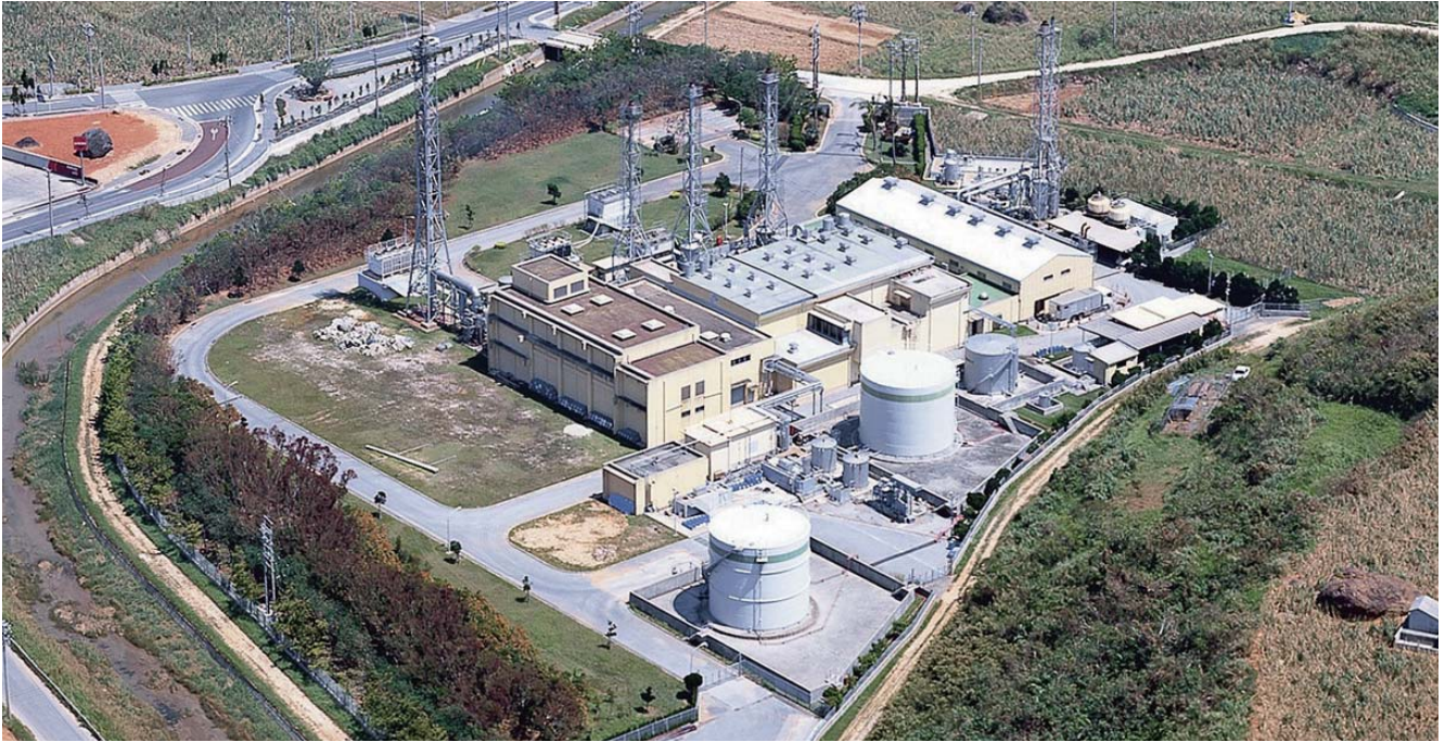
Kumejima power plant
