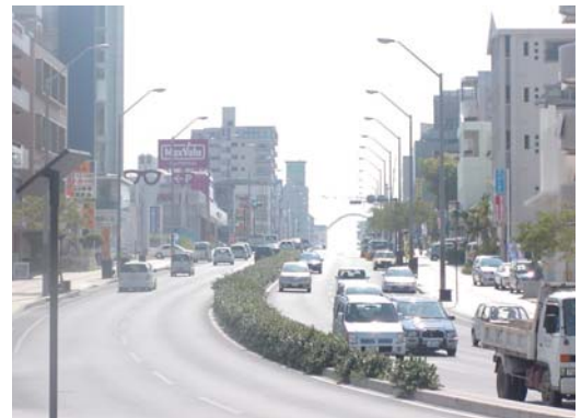
Street with underground power distribution lines
