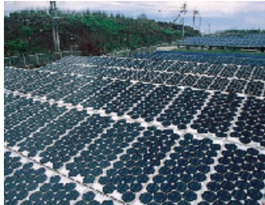
Photovoltaic Electric Power Generation System
