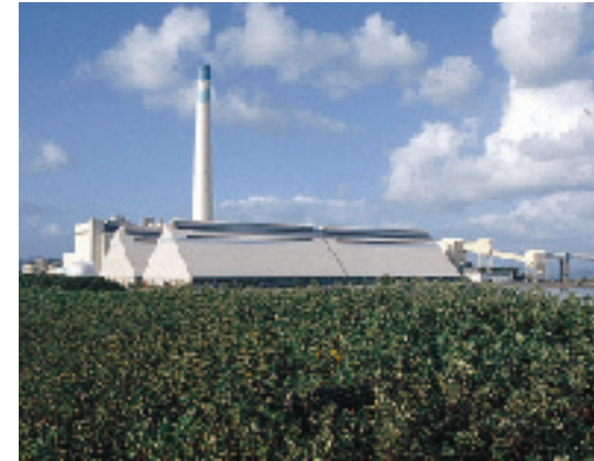
The Greening of Gushikawa Thermal Power Station
