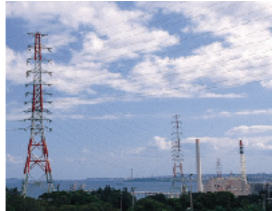
Increase in Efficient Transmission Facilities
