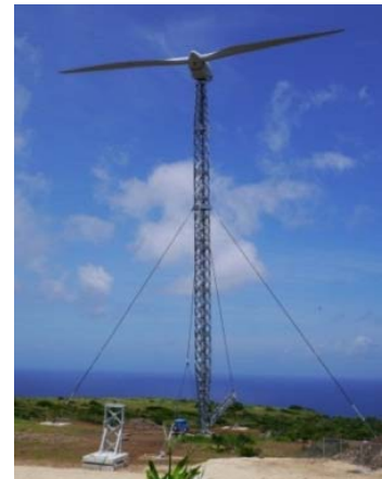
▲ Tiltable wind power generators ( Left picture : Aguni Island, Right picture : Hateruma Island )
