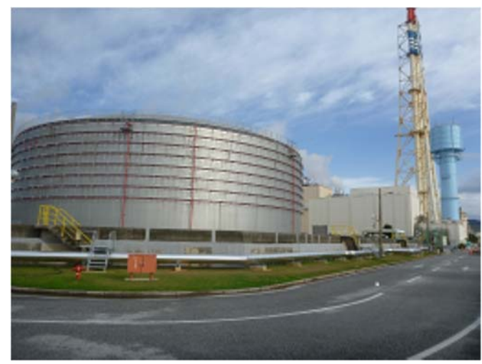
Heavy oil tank in Ishikawa Thermal
