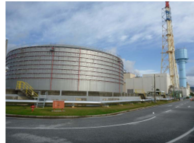
Heavy oil tank in Ishikawa Thermal (15,000kl)
