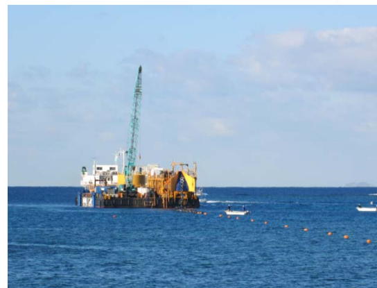
[Cable laying work with a special barge]
