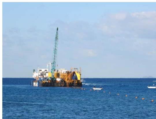
[Cable laying work with a special barge]
