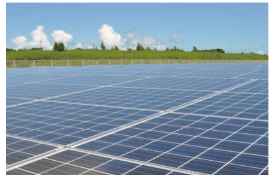
Solar power generation system on Tarama Island
