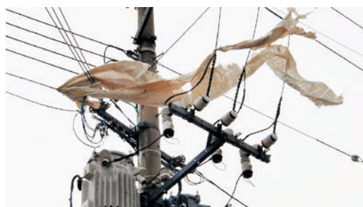
Damage due to flying debris
