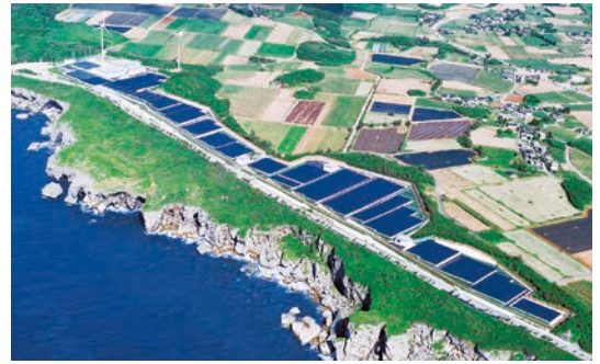
Solar power system on Miyako Island field test facility
