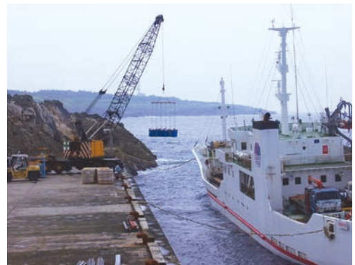
The transportation of fuel to Minami-Daito Island
