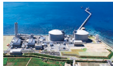
Yoshinoura Thermal Power Station
