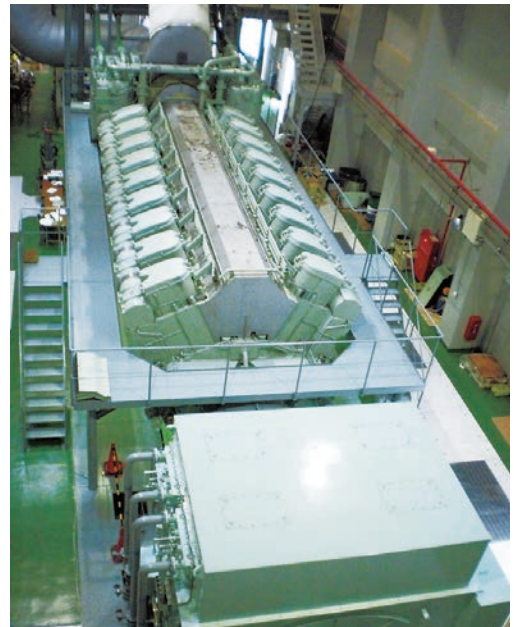
Ishigaki No. 2 Power Plant (diesel generator)
