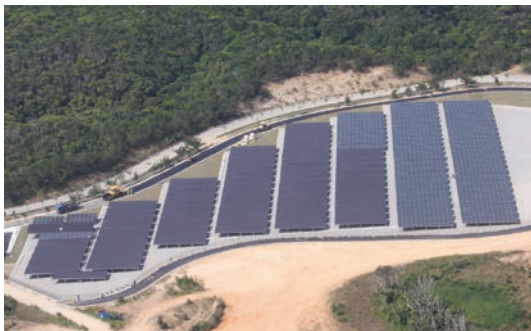
Abu Mega Solar Power Experimental Research Facility
