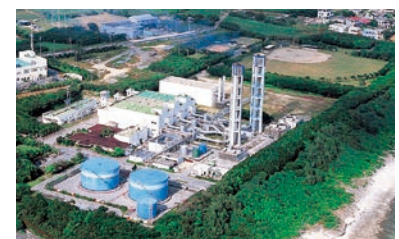
Green power plant (Ishigaki No. 2 Power Plant)
