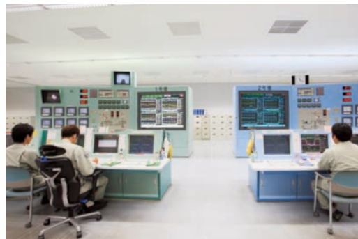
Kin Thermal Power Plant control room
