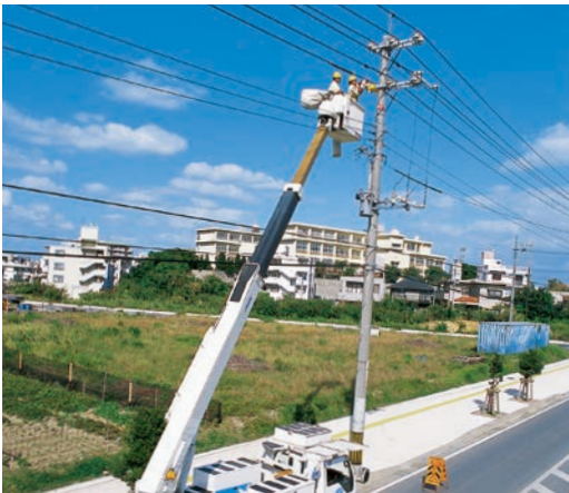
Distribution line maintenance
