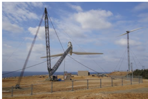
Retractable wind-power generator (Minami Daito Island)
