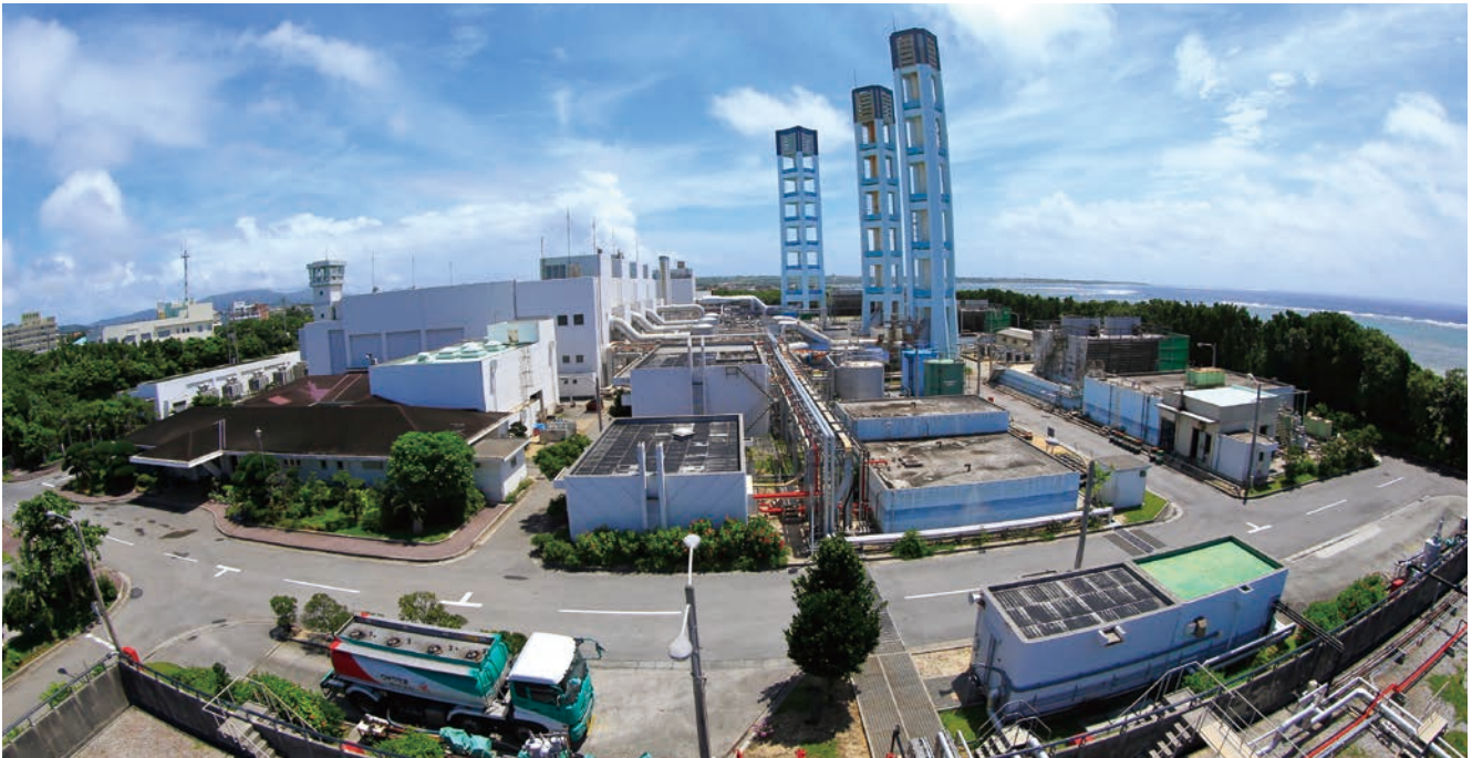
Ishigaki No. 2 Power Plant
