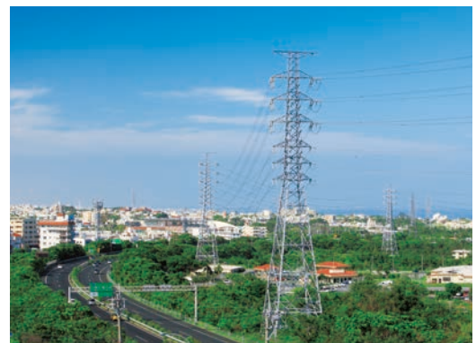
Transmission and distribution facilities
