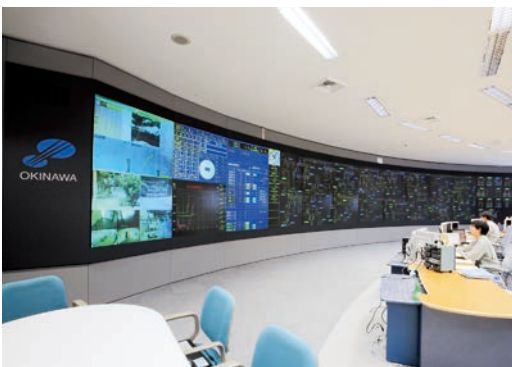
Load dispatching center
