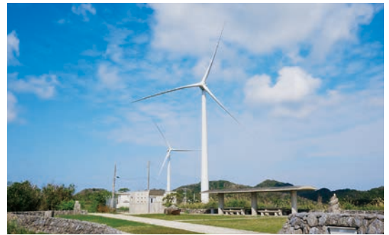
Ogimi Wind Power Generation Demonstration Research Facility
