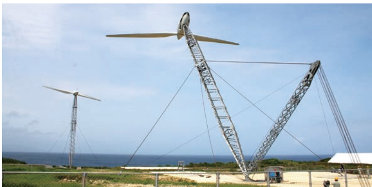
Retractable wind-power generator at Hateruma Island
