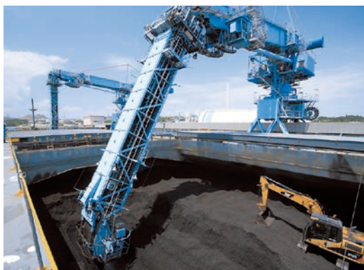
Unloading coal at Kin Thermal Power Plant
