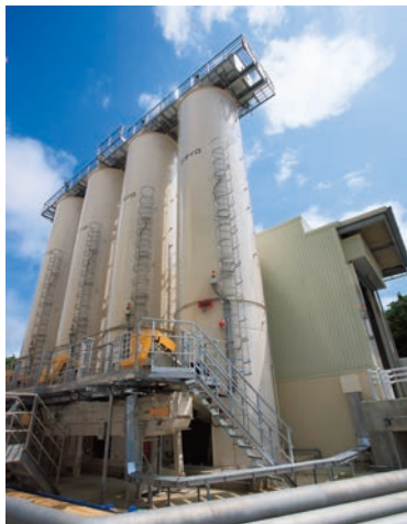
Biomass co-firing system
