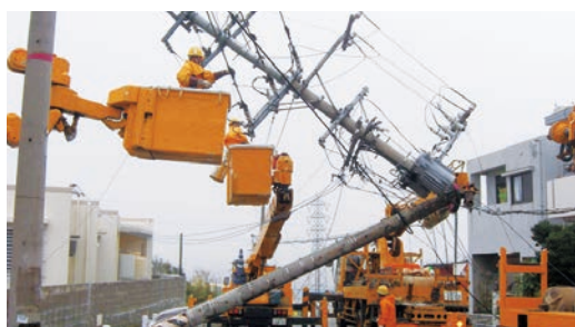
Electric power restoration operations
