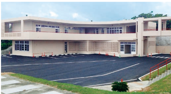
New building construction at Okinawa Christian School (Okidenko Co., Inc.)
