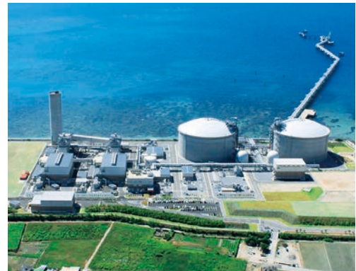
Yoshinoura Thermal Power Station
