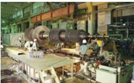
Staff from Okinawa Plant Kogyo Company, Limited disassemble a turbine at Makiminato Thermal Power Plant for a regular inspection.
