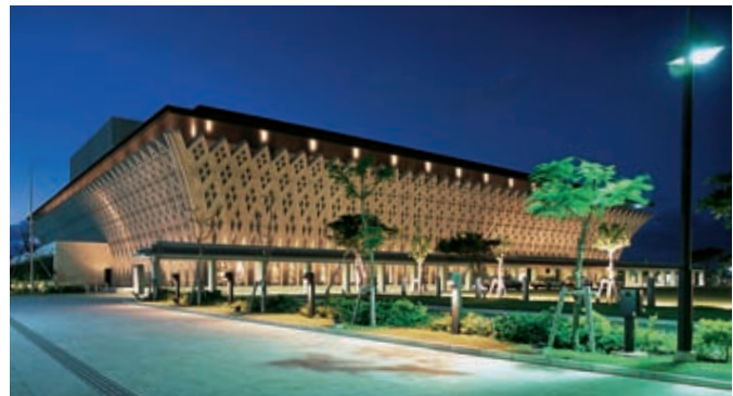
Okidenko Company Incorporated installed the exterior lighting for the National Theater Okinawa.
