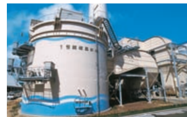
Environmental protection facilities at a power plant
