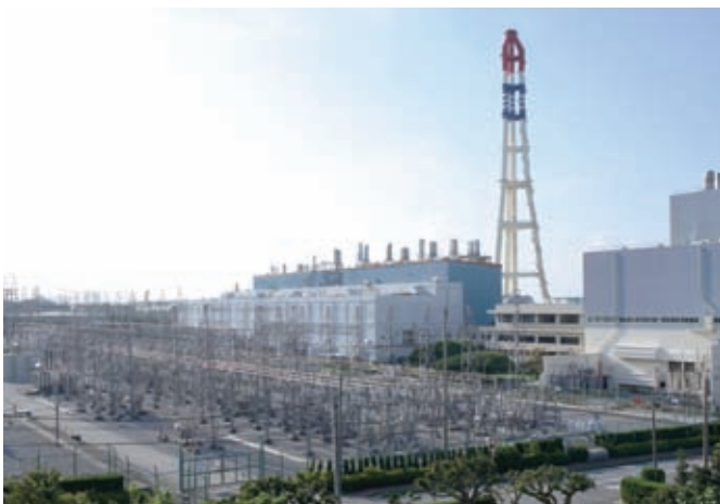
Makiminato thermal power station
