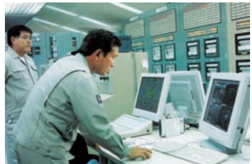
Remote monitoring of Miyako and Ishigaki power plants
