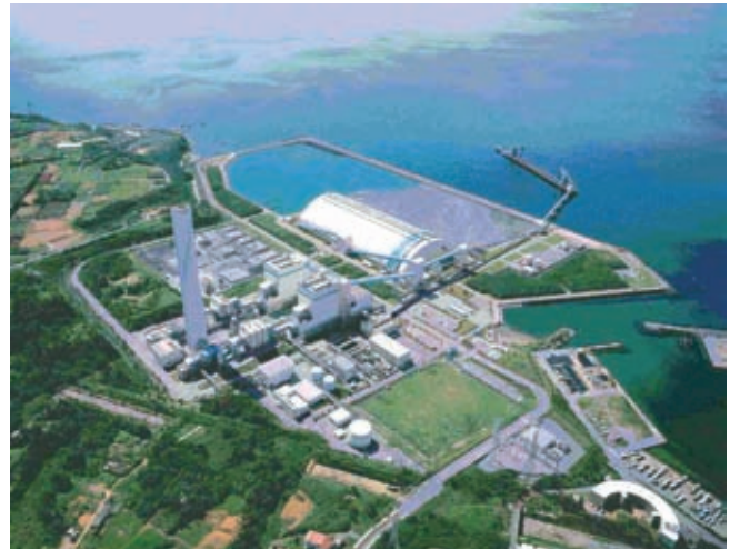
Kin thermal power plant
