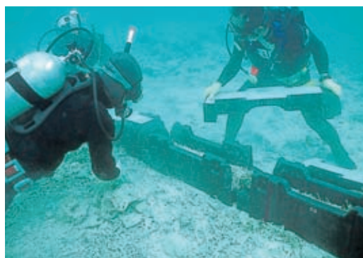
Submarine power cables
