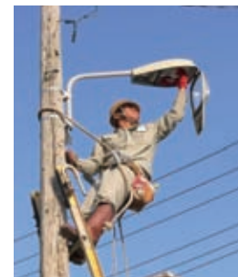
OEPC employees inspecting street lights
