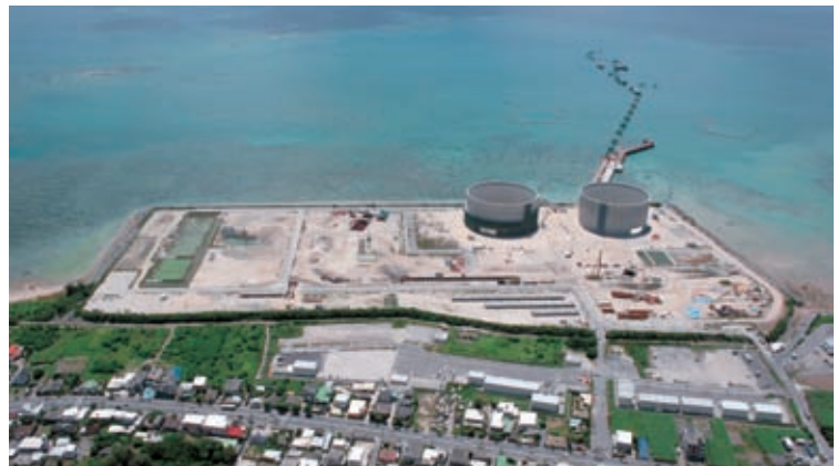
Yoshinoura thermal power plant during construction
