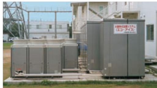
Ice-storage air conditioning systems
