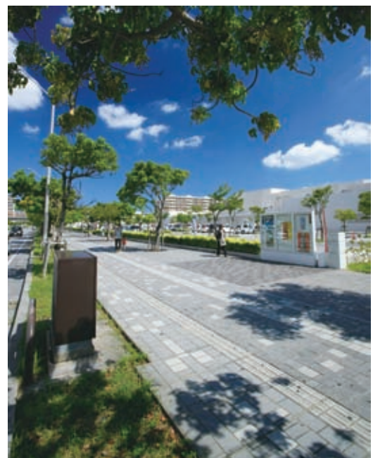
Street with underground power distribution lines
