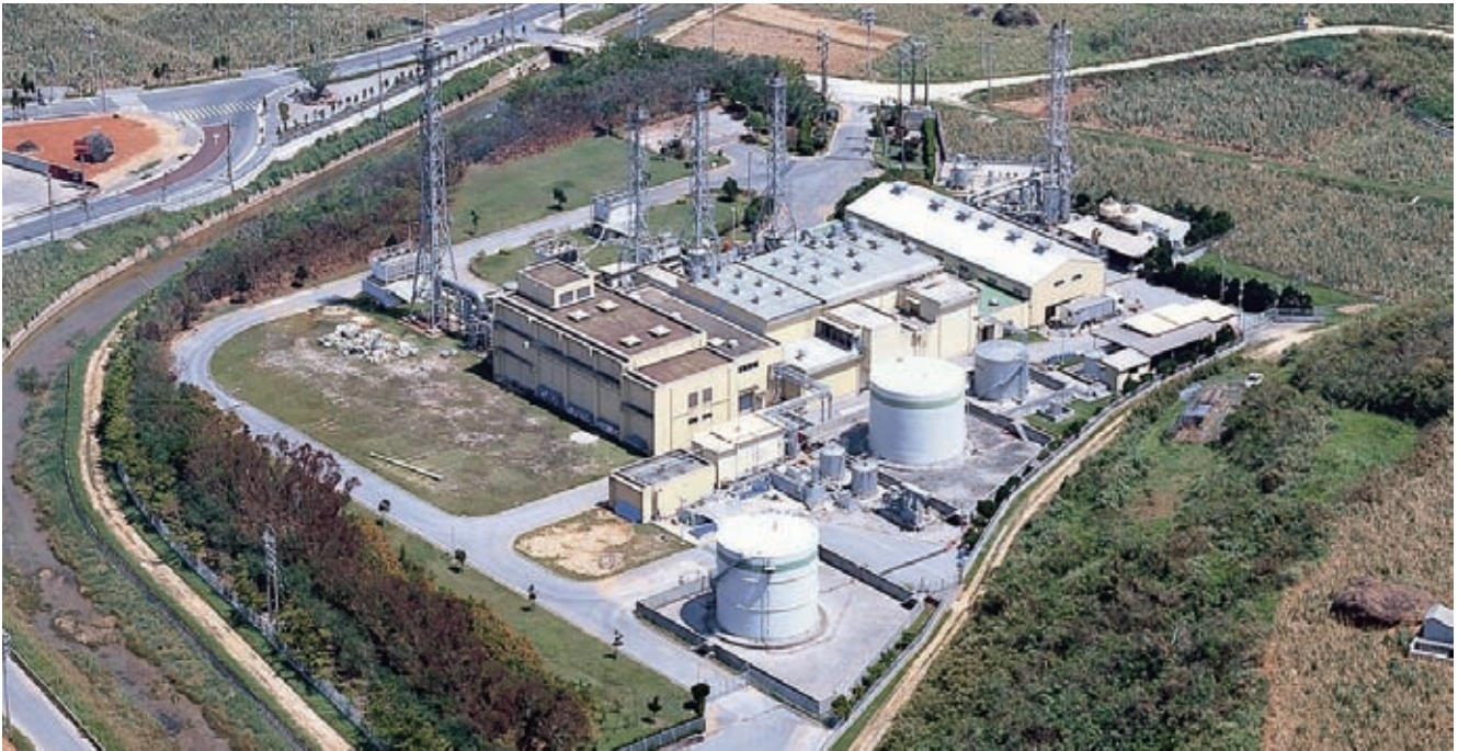
Kumejima power plant
