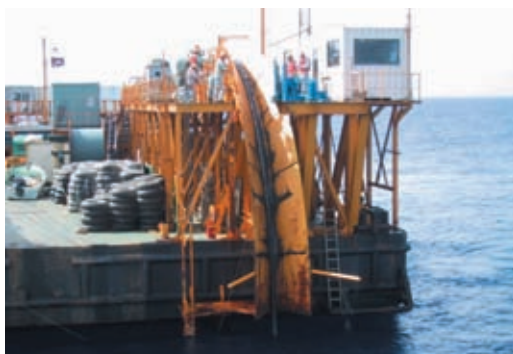
Laying submarine power cables
