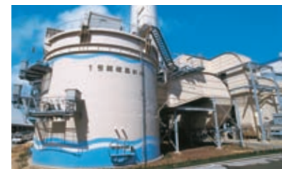
Environmental protection facilities at a power plant
