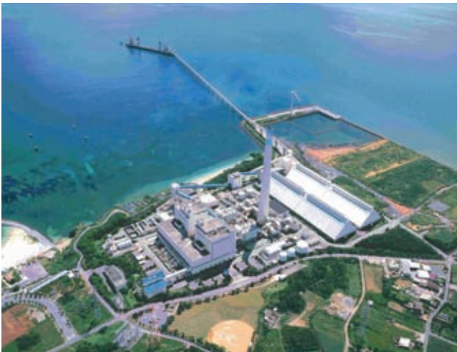
Gushikawa thermal power plant
