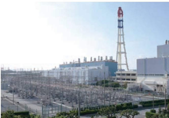
Makiminato thermal power station
