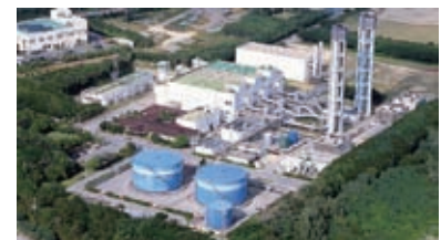
Ishigaki No. 2 Power Plant (diesel turbine plant surrounded by 90,000 native trees planted by the Company)
