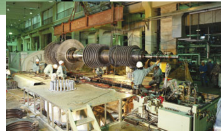
Staff from Okinawa Plant Kogyo Company, Incorporated disassemble a turbine at Makiminato Thermal Power Plant for a regular inspection.
