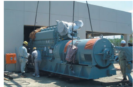
Installing a small-scale power generator
