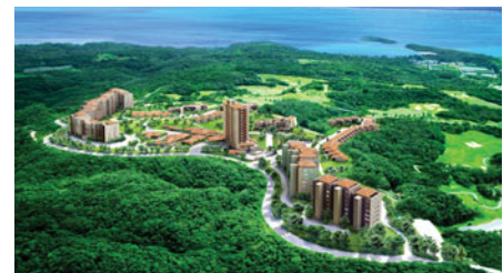
Artist's impression of the Kanucha Community, a retirement community complex with nursing care facilities
