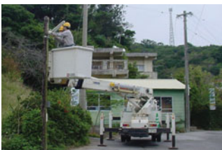
OEPC employees inspecting street lights
