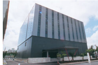
The iDC Building — This building features highly reliable broadband Internet access services, provided by First Riding Technology Company, Incorporated.
