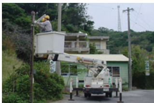
OEPC employees inspecting street lights
