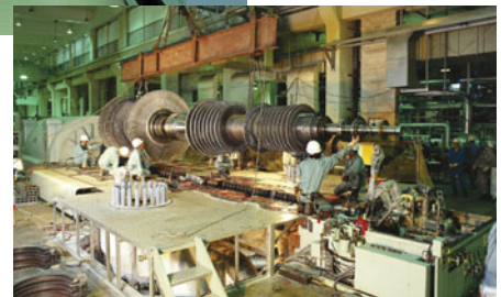
Staff from Okinawa Plant Kogyo Company, Incorporated disassemble a turbine at Makiminato Thermal Power Plant for a regular inspection.
