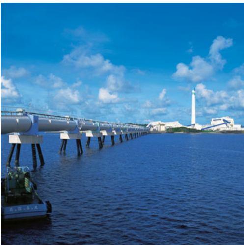
Gushikawa Thermal Power Station
