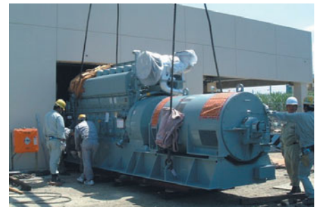
Installing a small-scale power generator
