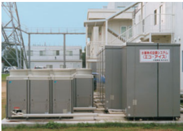
Ice-storage air conditioning systems
