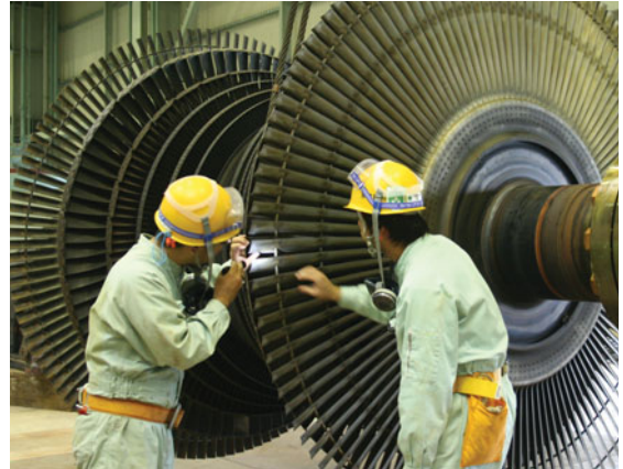
Power generation turbine
