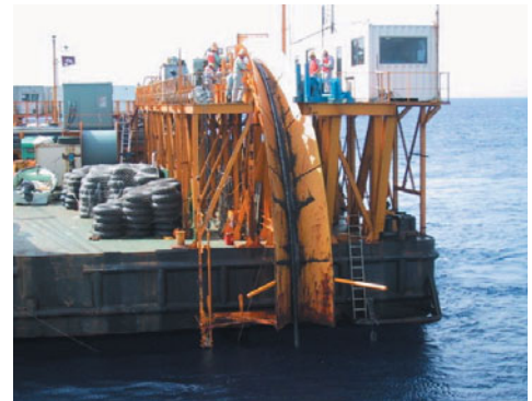
Laying submarine power cables
