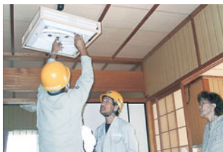
Checks and repairs on wiring in homes where elderly people live alone
