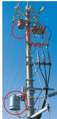
Automatic power distribution monitoring system
