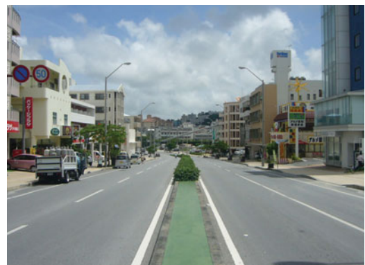
Street with underground power distribution lines
