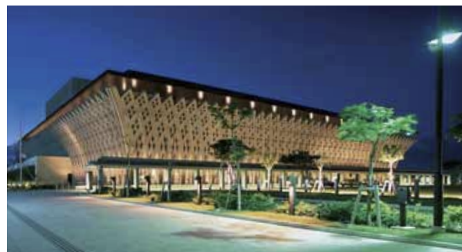
Okienco Company Incorporated installed the exterior lighting for the National Theater Okinawa.
