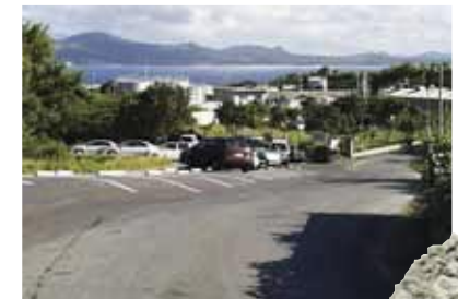
Road surfaced with OEPC's Pozotech
