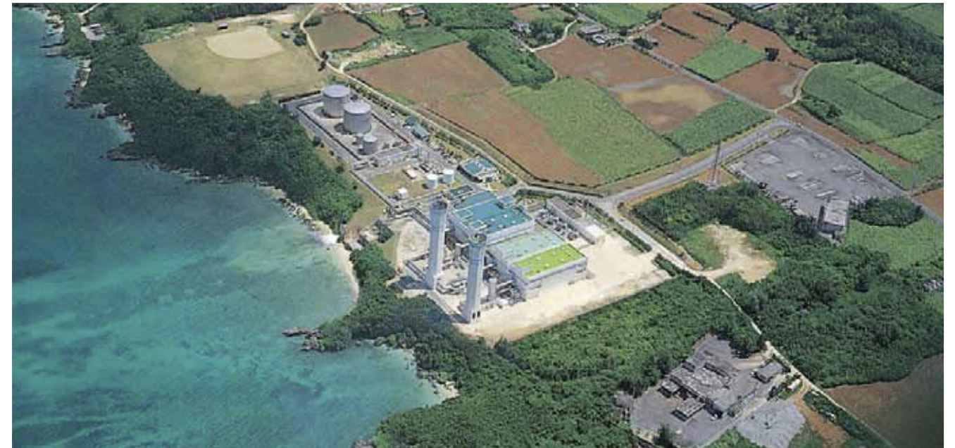
Miyako No.2 Internal Combustion Power Station
