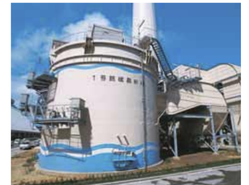
Environmental protection facilities at a power plant As part of an overall policy of removing harmful chemicals from smoke emitted by our power plants, they are equipped with desulphurization and denitrification equipment.
