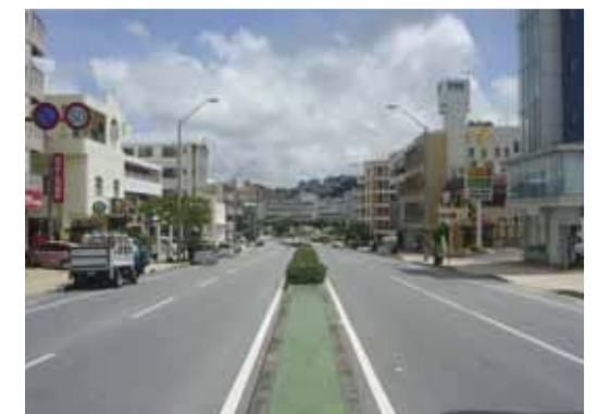
Street with underground power distribution lines
