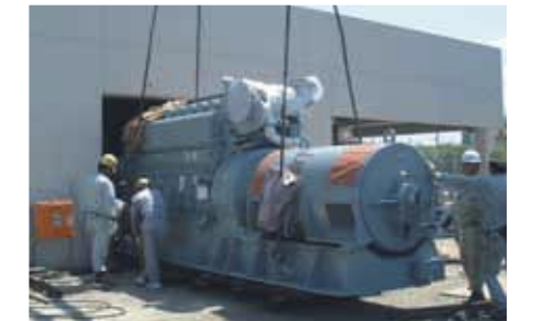
Employees of Progressive Energy Corporation (PEC) install a small-scale power generator, part of a "distributed generation" network.
