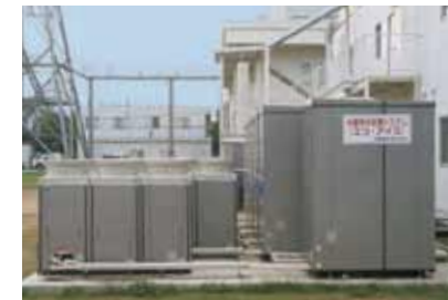
Ice-storage air conditioning systems
