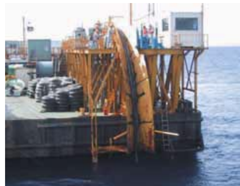
Laying submarine power cables
