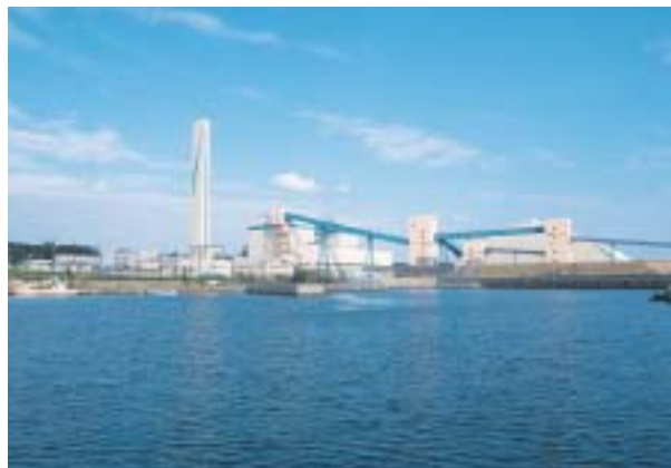
Kin Thermal Power Station
