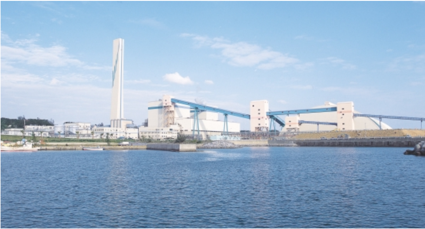
Kin Thermal Power Station
