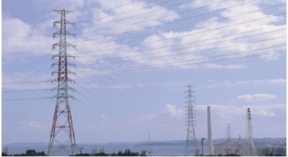
Power transmission route
