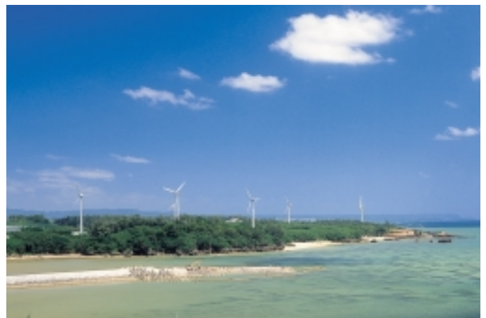
The Ginoza Wind Power Research Facility
