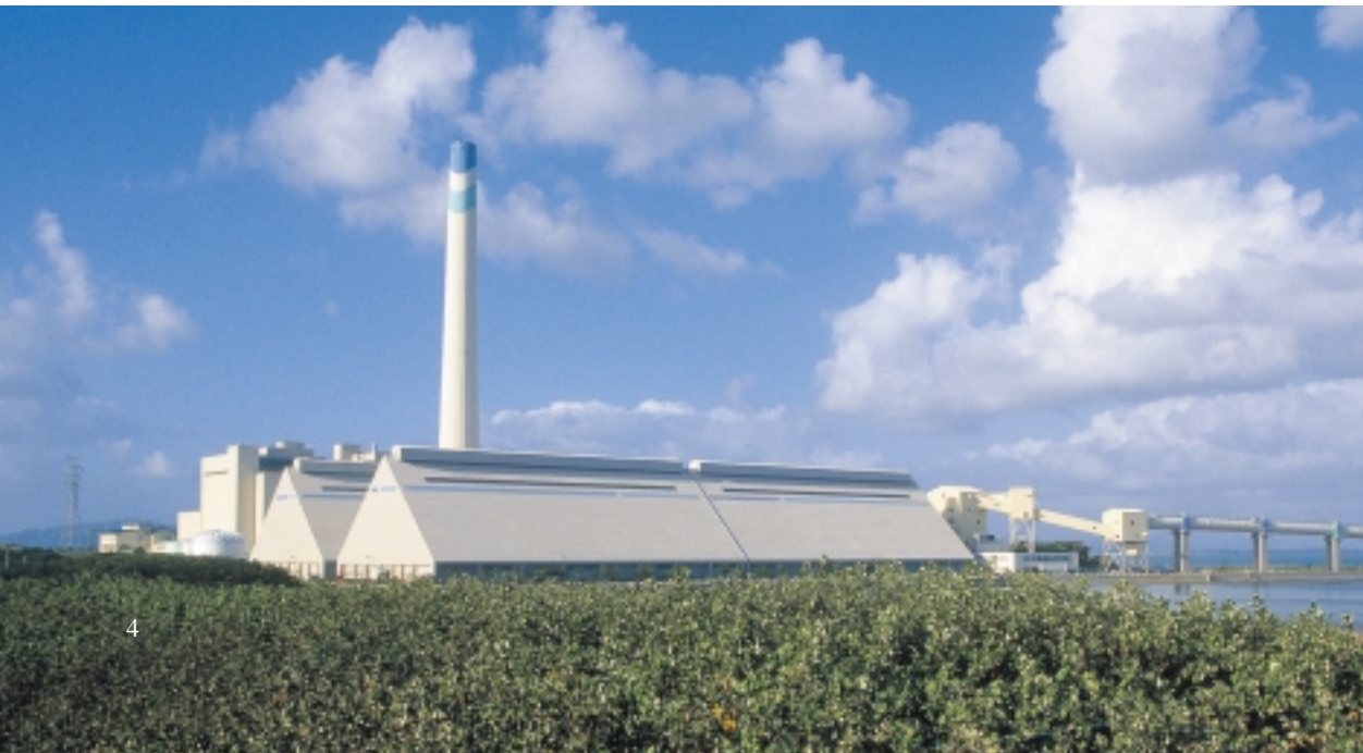
Gushikawa Thermal Power Station
