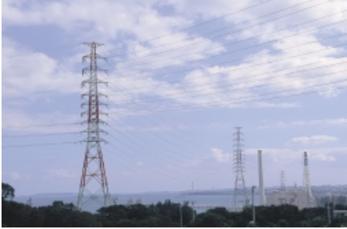
Power transmission route
