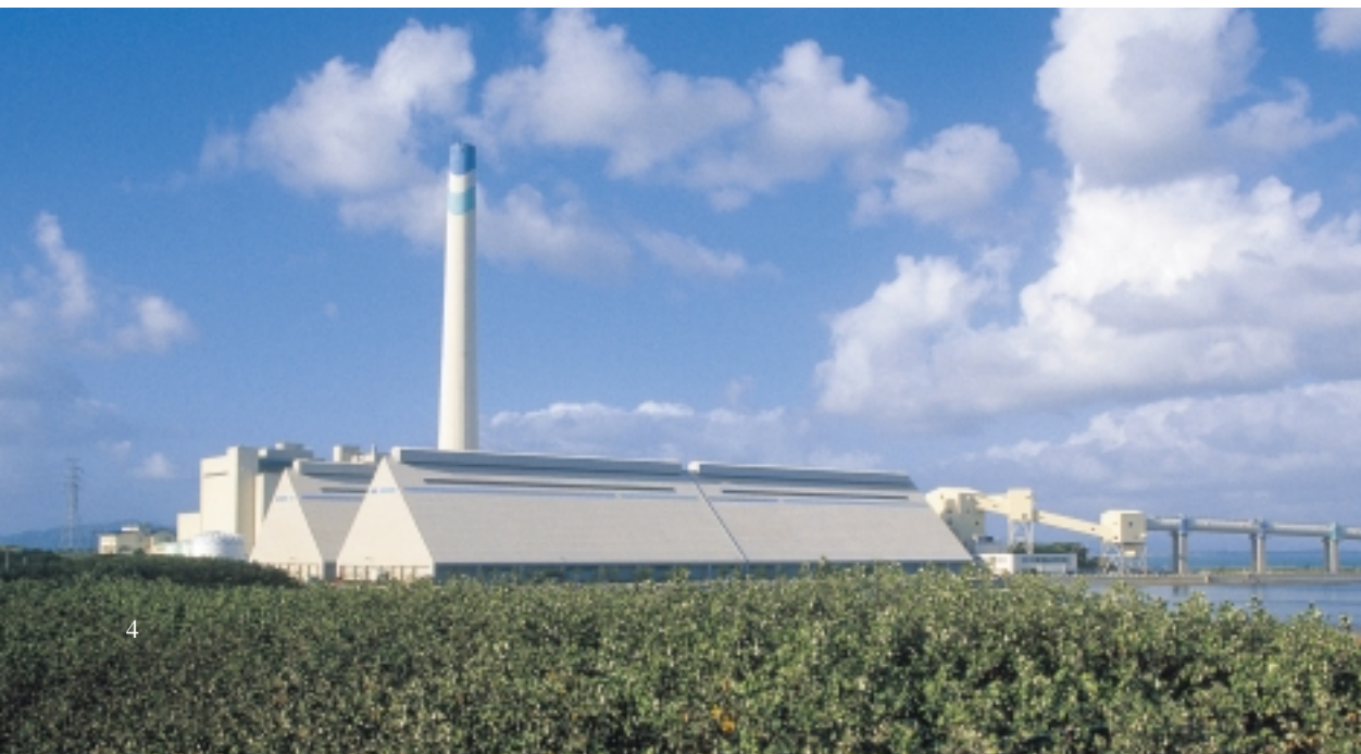
Gushikawa Thermal Power Station
